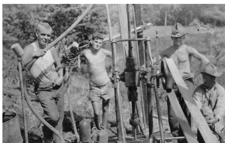
Diamond drill crew at Miramar lock site, December 18, 1930. Diamond drills were used to obtain rock strata samples.
