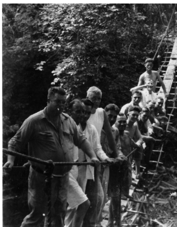
A suspension bridge over the Rio Grande River at Camp Deakne, constructed by the battalion's Company A.
