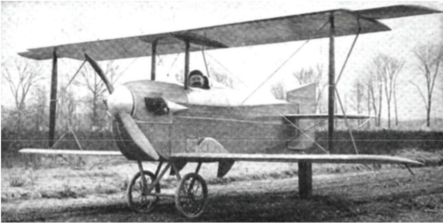
Martin's K-III scout aircraft incorporated several of his patented devices: K-bar Strut (US 1,277,979, 1916), Retractable Landing Gear (US 1,306,768, 1916), and Shock Absorbing Rudder (US 1,464,209, 1918).
