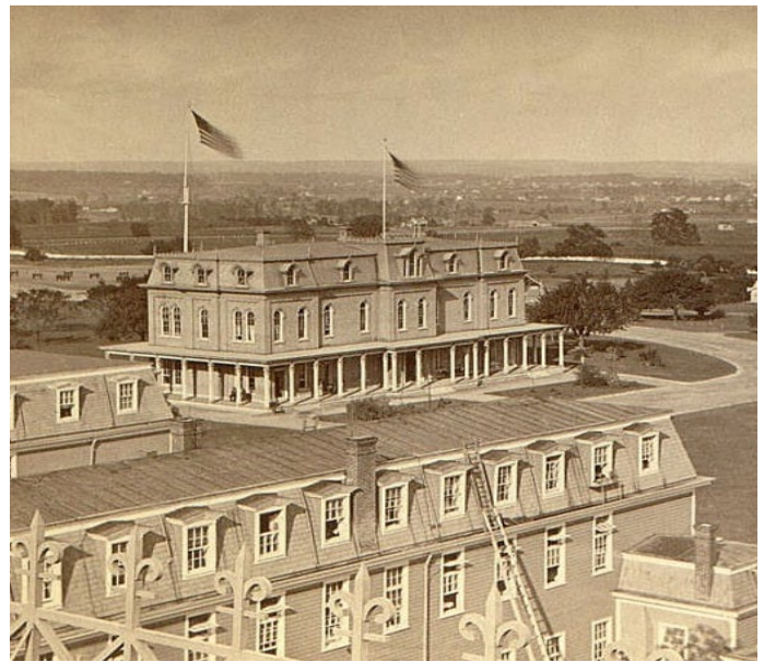
Old headquarters building at the VA Medical Center campus in Dayton, OH, and future home of the National VA History Center.
